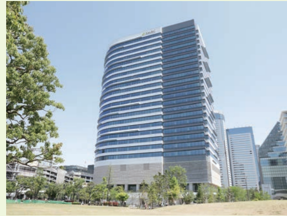
Exterior of Headquarters Office
